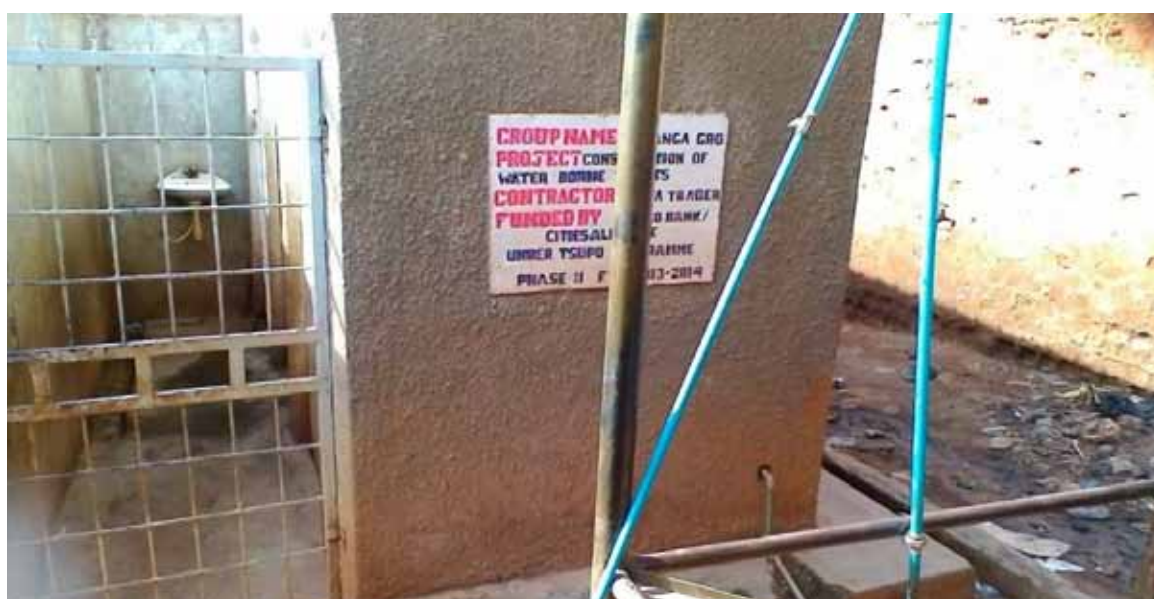
Figure 24 A Water-borne Toilet in Industrial Division, Mbale
