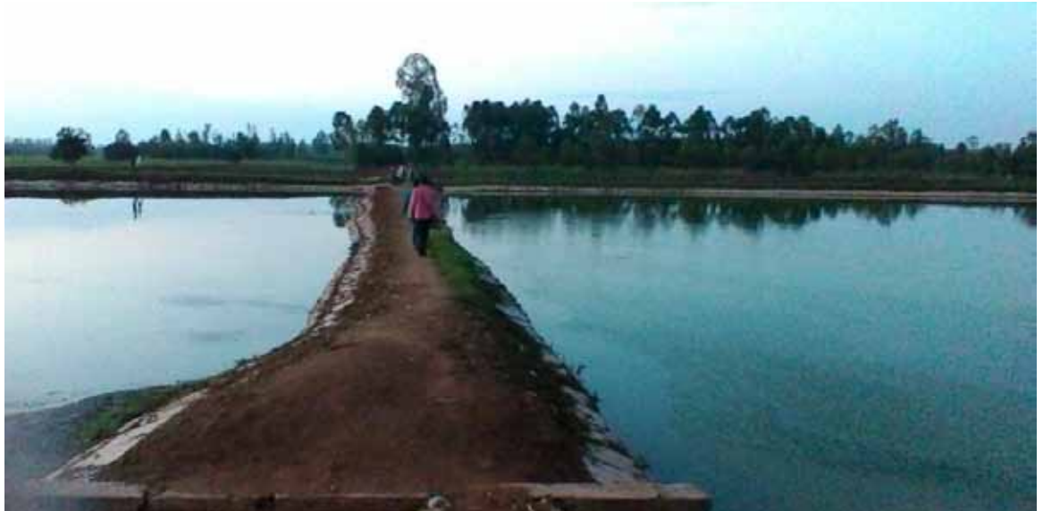
Figure 26 Lagoons for Liquid Waste Collection in Industrial Division, Mbale
